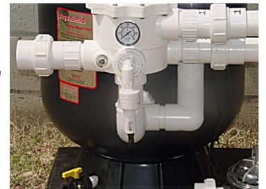
After double checking all connections to make sure they are tight you are ready to prime and start the system. We recommend that a "SWING" check valve be installed below surface grade of pond on intake into the system. This will make the priming of the system a snap. To Prime system, fill AquaSieve (if so equipped) with water and pump with water. Close the units and start pump.
