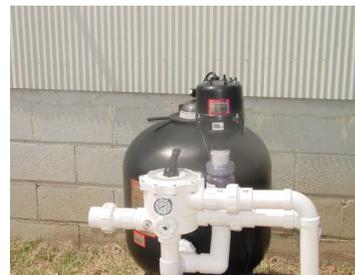
Step 9: Place Bead Agitator onto AquaBead filter. Note: Do Not Glue. Normally pressure fitting into place is sufficient. If it isn't, secure with a set screw through Agitator into pipe.
