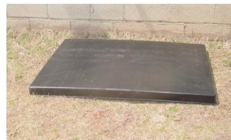
**Step 1: Start by laying the Pad(s) on level ground where you want to locate the equipment.**
