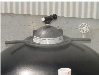
Note: Make sure no beads are on or in the threads before installing and tightening.
