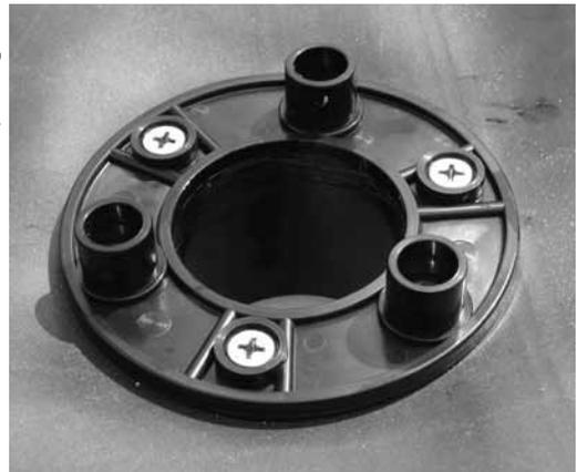
**6** Once the halves have been securely joined, carefully cut away the circular portion of the liner inside the drain, making sure to trim the liner flush with the inside edges of the drain. Apply a light coating of silicone sealant to the inside surface of the drain.
