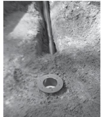
**4** Install your 45 mil EPDM liner. After your liner is fully installed, locate the spot where the lower half of the bottom drain has been installed underneath the liner, using your fingers find the six screw holes located in the gasket and rim of the bottom drain lower half. With a white pencil mark your liner with the loca-
