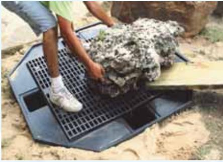
Carefully set feature in center of grating. Align hole in feature with hole in grate. It may be necessary to drill a larger hole in the grating to accommodate bigger tubing.
