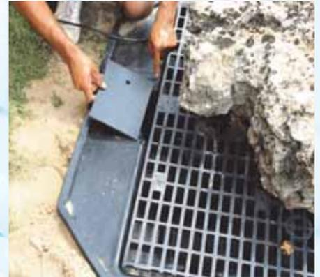
Place lid over pump compartment. Spread decorative gravel or river rock on grating, just enough to cover grating is all that is required. You can easily remove the pump anytime by clearing the gravel or river rock off lid. Fill basin with water and plug pump into a GFI protected outlet with weather cover.
