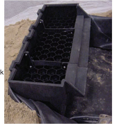
The liner goes under the spillway and wraps up the back and ends.
